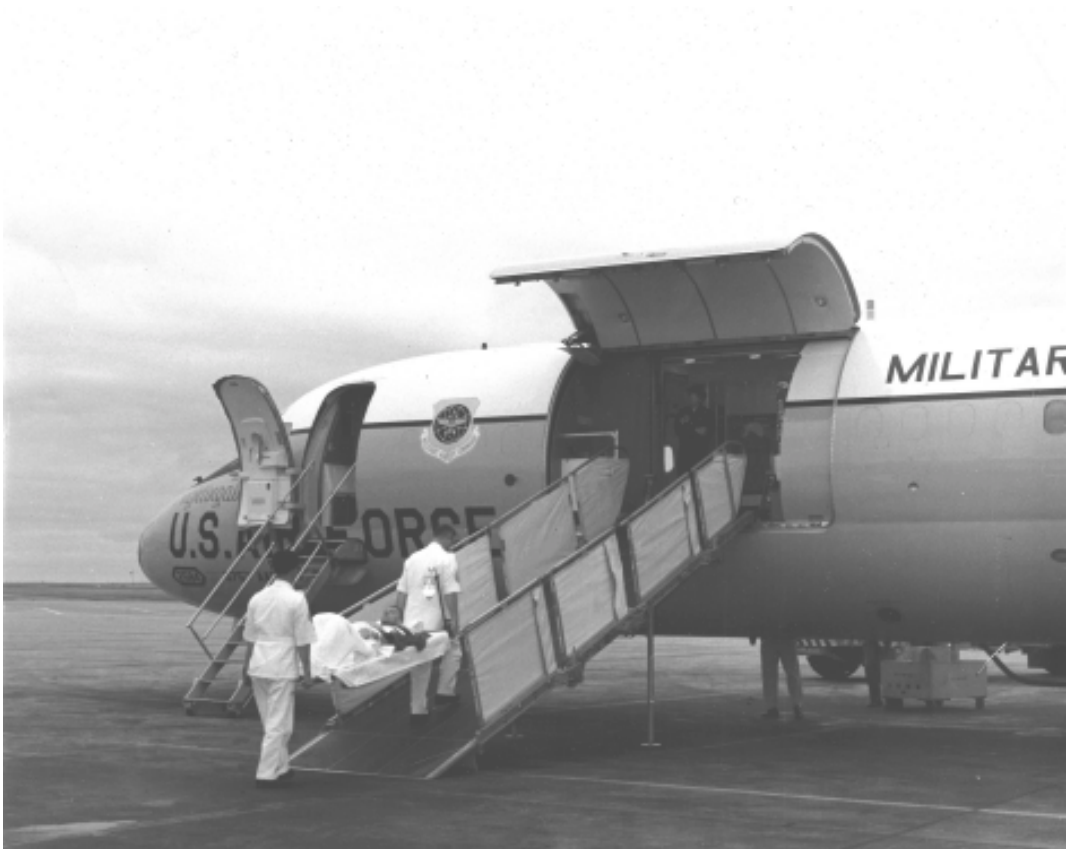
Medical personnel carry a litter patient up the C-9A's hydraulically operated folding ramp, a feature unavailable on commercial aircraft.
