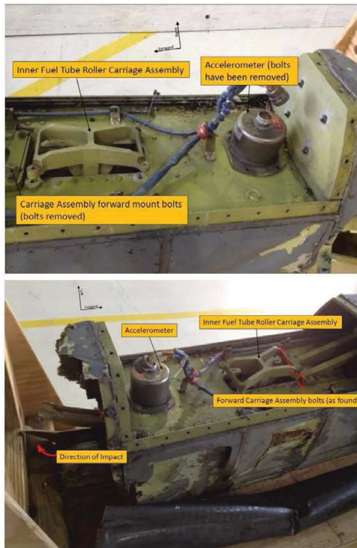
Figure 2. Condition of accelerometer and surrounding structure during SIB teardown.
