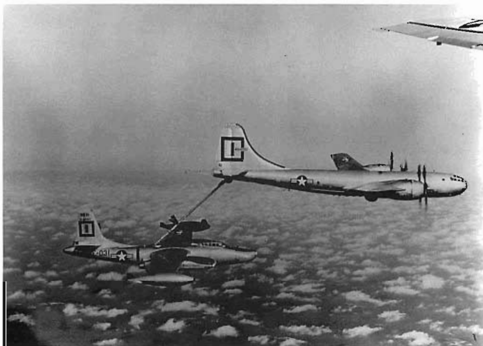
A KB-29P assigned to the 91st Air Refueling Squadron, Barksdale Air Force Base, Louisiana, puts Strategic Air Command's long reach into practice by refueling an RB-45C, which was assigned to the 91st Strategic Reconnaissance Wing.
