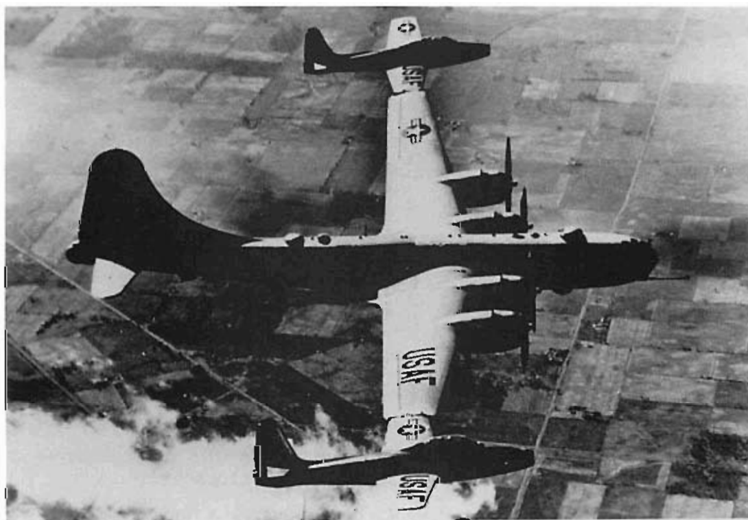
Prior to developing inflight refueling for fighters, the Air Force experimented with ideas such as "Project Tip-Tow," which investigated the towing of aircraft like these two F-84s by bombers such as the B-29.
