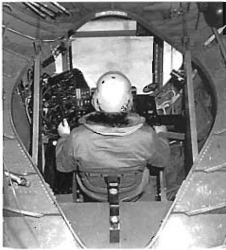
Boomer at work--unlike his predecessors in the KB-29, the boomer in the KC-97 was able to sit upright while working the aircraft's flying boom.
